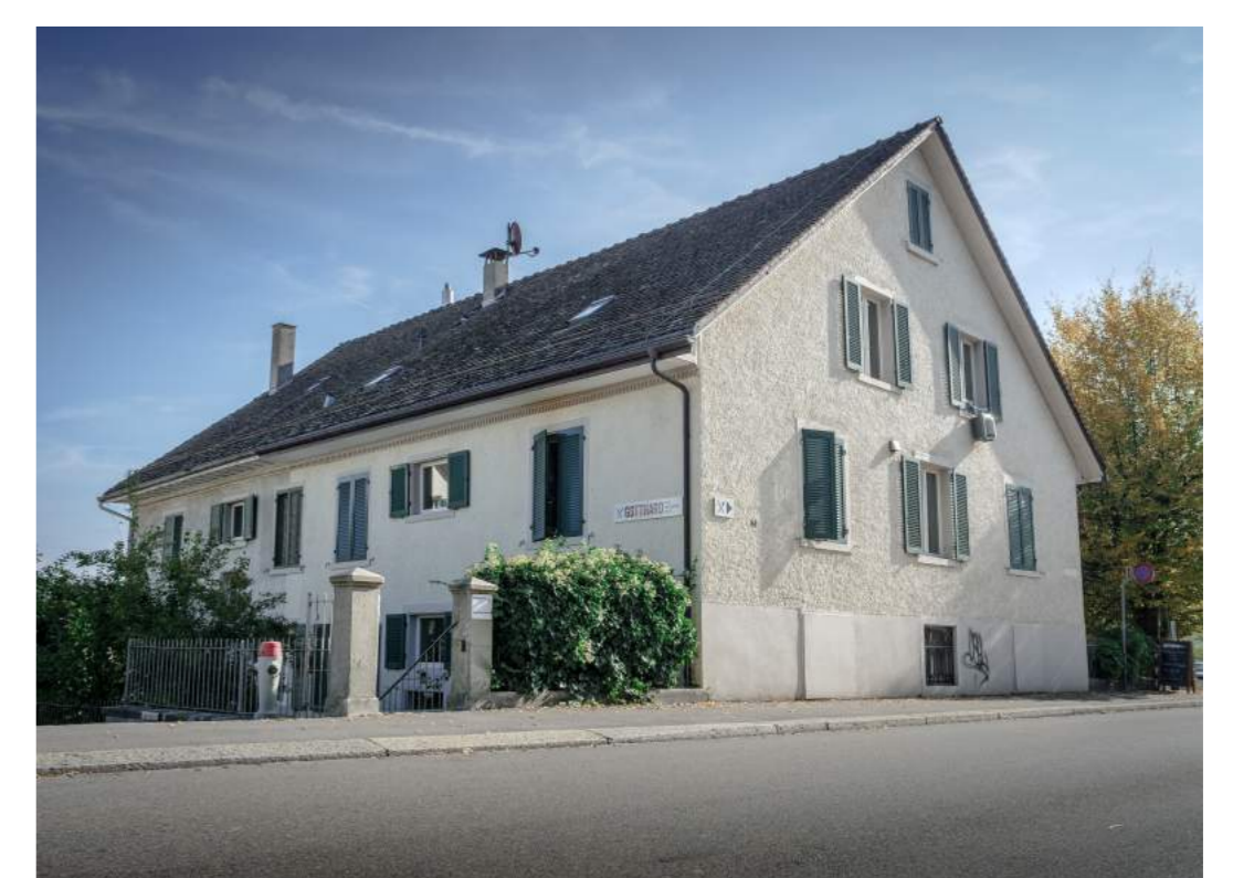
Gotthardstrasse 2a, Thalwil
